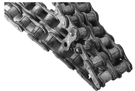
Fig. 31 Corrosion of stainless steel roller chain
